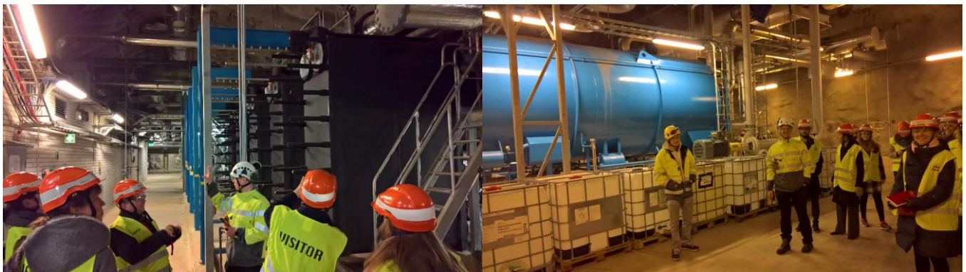
Visit of underground cooling station – seawater exchangers and absorption chiller
