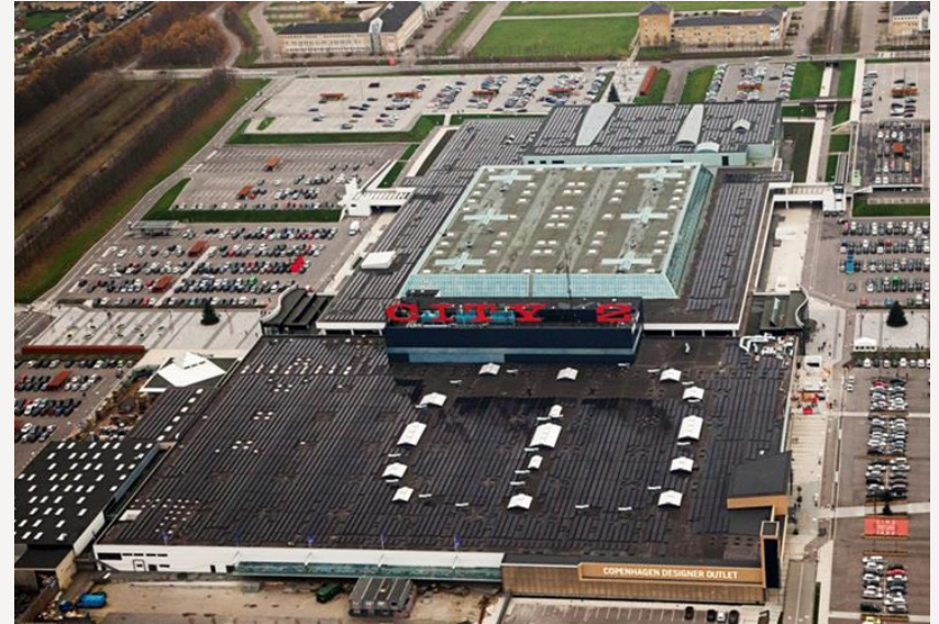
16,200 m 2 PV on the roof (2.1 MWp)
