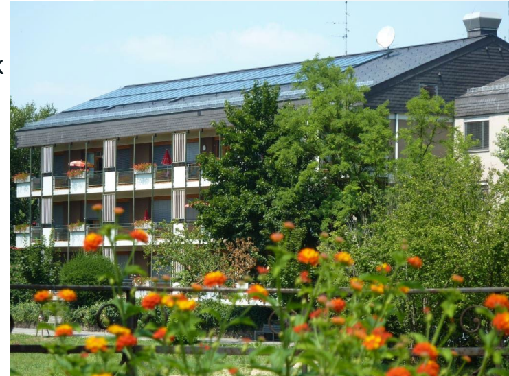
Elderly home post IEC - Bad Radkersburg, Styria, Austria Source: Landesimmobiliengesellschaft Steiermark GmbH
