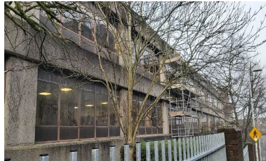
Food Science Block B Retrofit – HEA Pathfinder 3 supported
